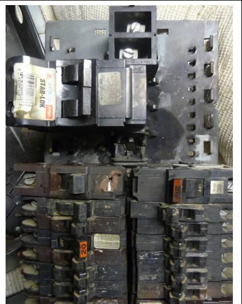
Fig. 3. Stab-lok® Breakers
