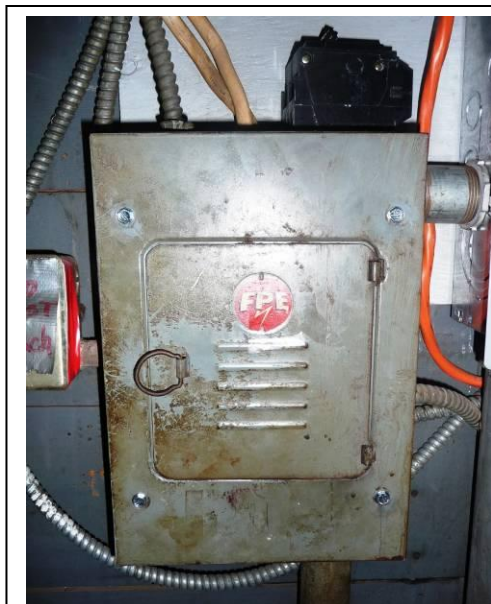
Fig. 1. FPE Stab-lok® Small Panel Box
