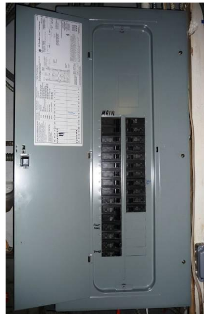
Fig. 12. New Replacement Panel Photo courtesy SCM Engineering, © 2012. Used with permission.
