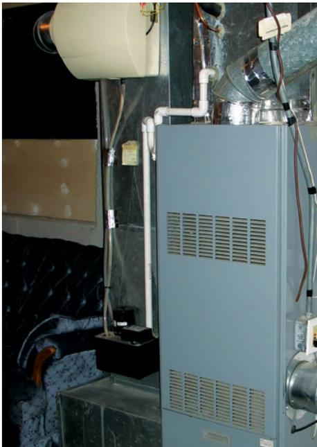
*Photo: A condensate pump can be seen in the lower left of the photo. © Big Stock Photo.*
