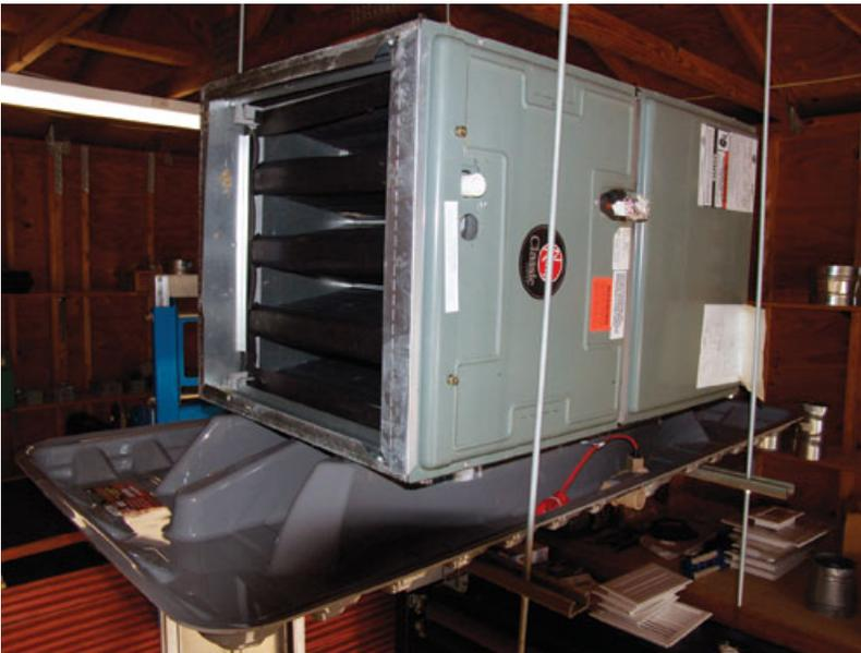
*Photo: Manufactured auxiliary drain pans, like the one in the photo, hold the air handler or furnace above the overflowing condensate. This is important as it can prevent damage to the equipment and make the pan easier to clean. Photo courtesy Resource Conservation Technologies, makers of AquaGuard brand HVAC accessories.*
