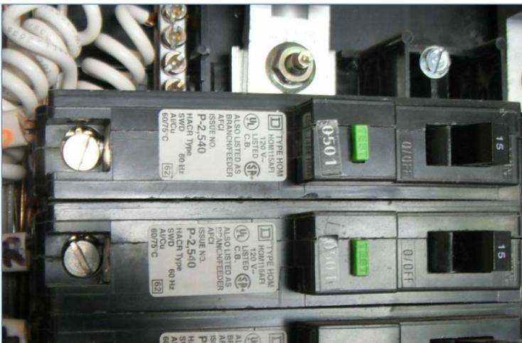
Figure 2 Branch/Feeder AFCI Label
